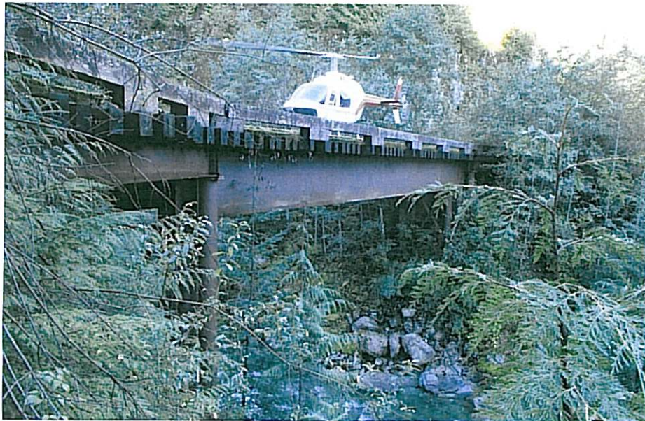
CK-2230 From downstream
